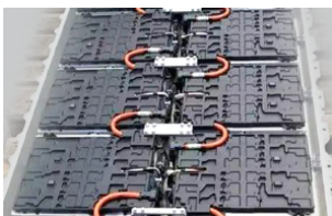
Battery charge/discharge test
